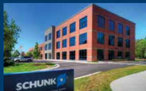
Plant Morrisville, USA SCHUNK Intec Inc. 211 Kitty Hawk Drive Morrisville, NC 27560, USA Tel. +1-919-572-2705 info@us.schunk.com
