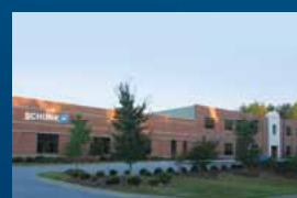
1992 Morrisville plant, NC USA
